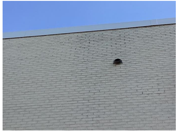
Eroded Mortar
