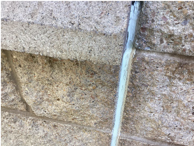
Dried and missing flexible sealants
