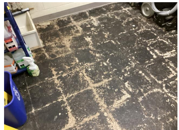
Tiles Removed, Suspect Mastic Exposed
