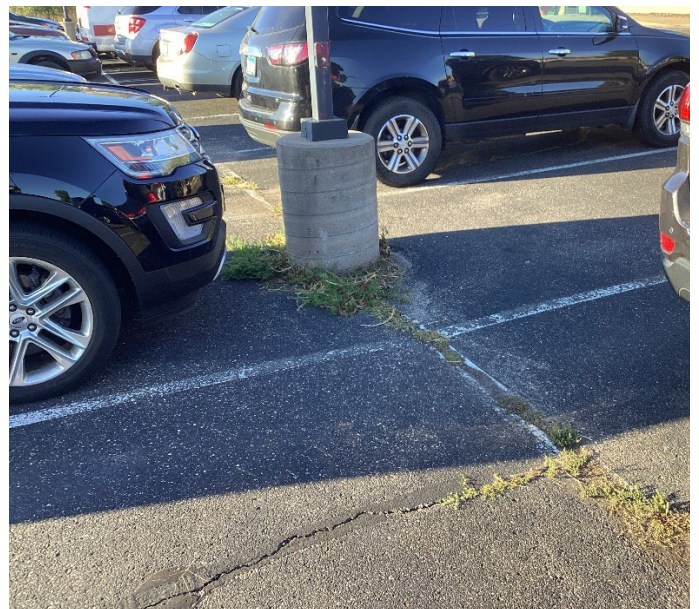
Cracked, settled, and dry pavement
