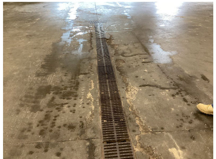
Damaged concrete in main shop
