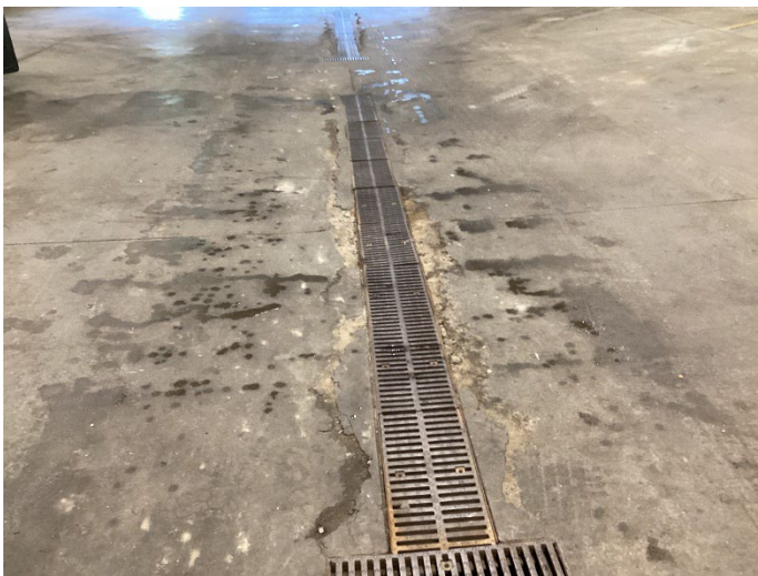
Damaged concrete in main shop
