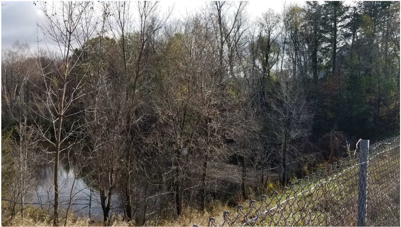
Photos: Outlet Control Structure pictured from Lofton Ave
