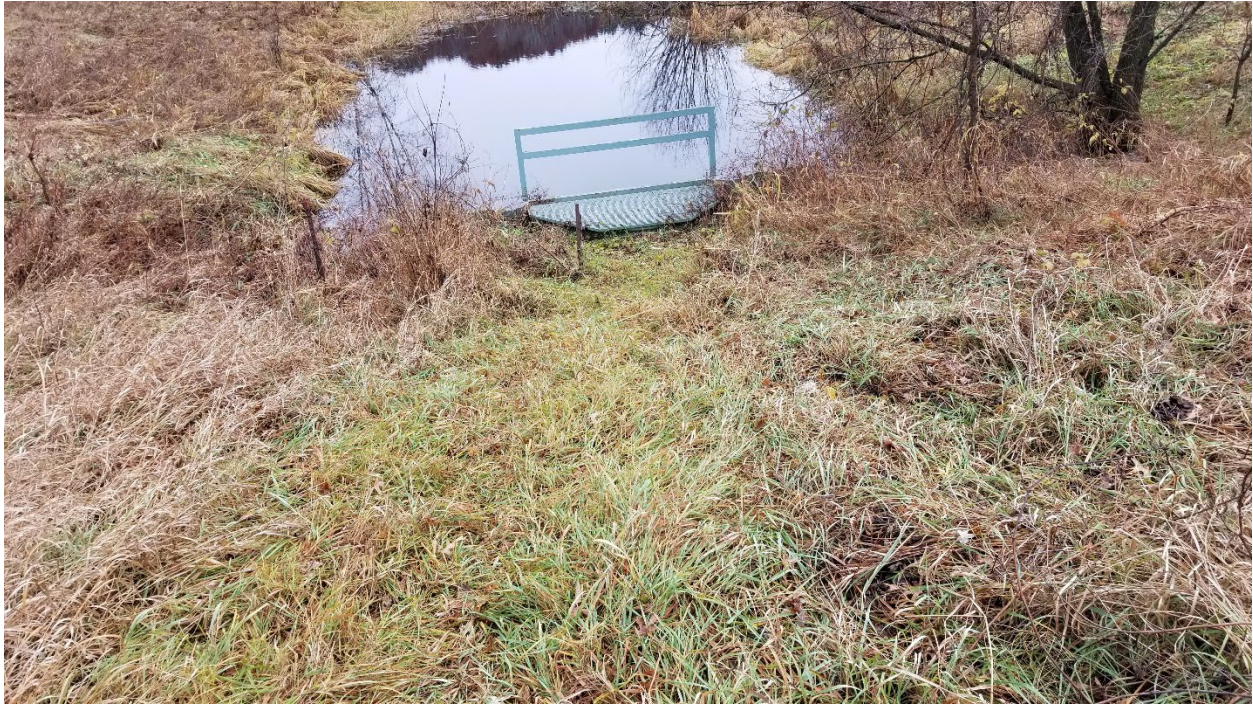
Photo: Channel upstream of Ivywood Control Structure
