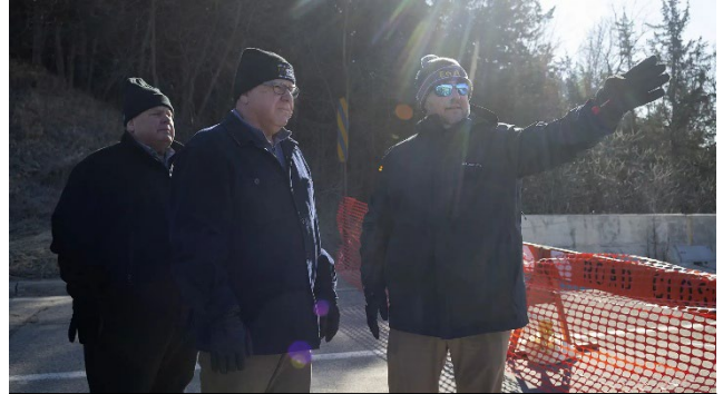
Shout out to Blue Earth County, including Commissioner Kevin Paap (left) and County Engineer and Public Works Director Ryan Thilges (right), who were featured at the governor's announcement and received a recommendation of $10 million for removal of the failed Rapidan Dam.
