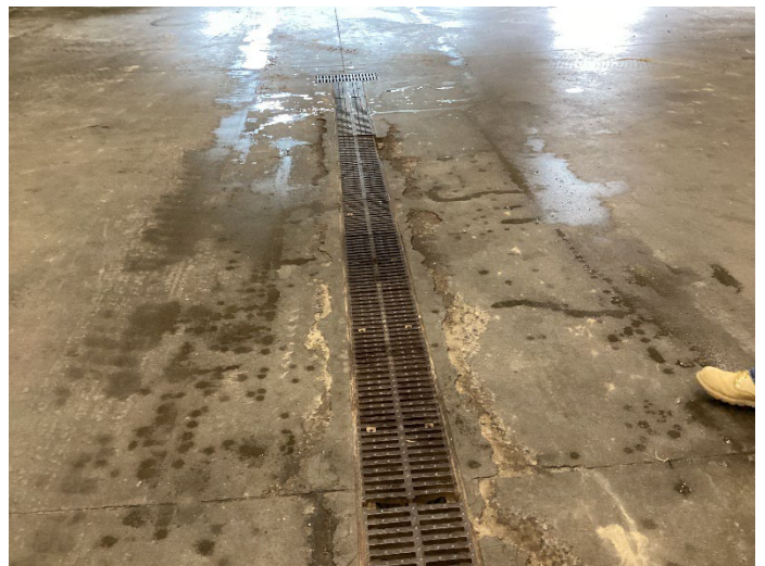
Damaged concrete in main shop
