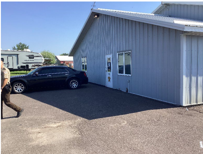
Poor drainage and elevation of front door
