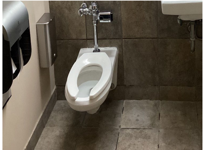
Damaged tile and missing tile grout
