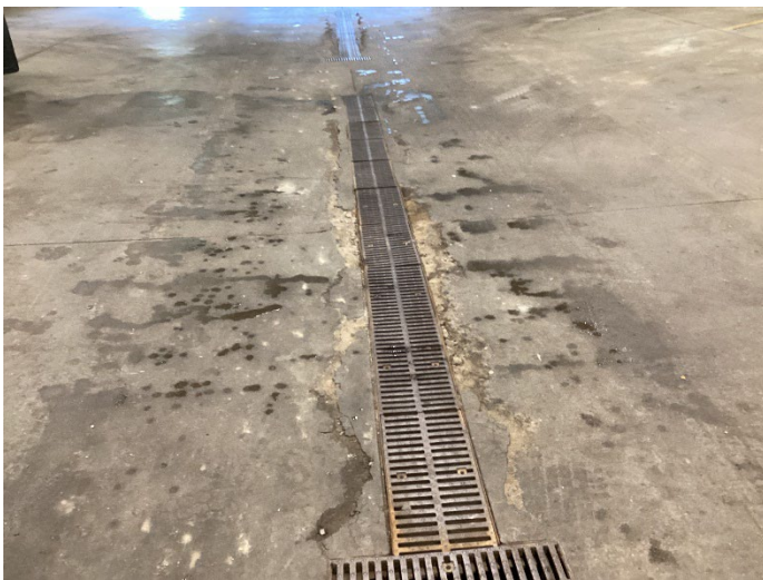
Damaged concrete in main shop
