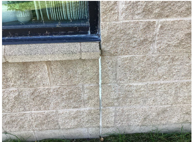
Dried and missing flexible sealants
