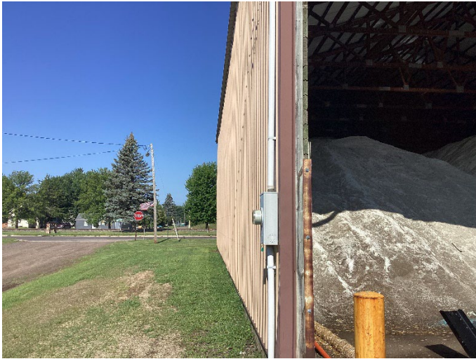
Bowing exterior walls
