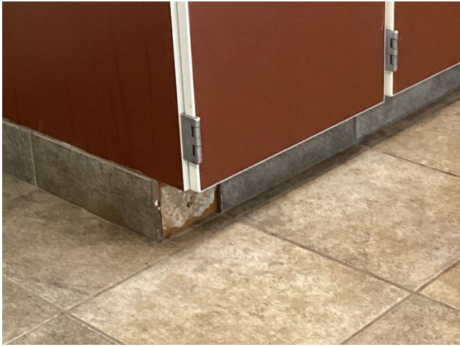
Damaged tile and missing tile grout
