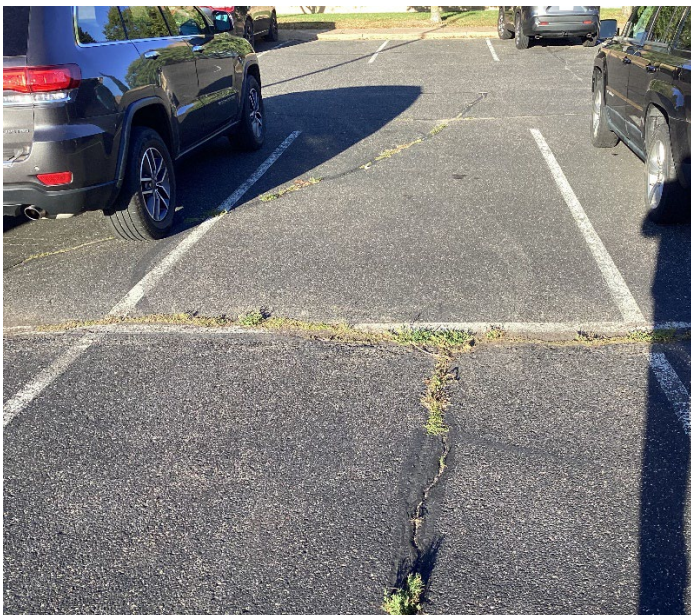
Cracked, settled, and dry pavement
