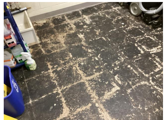
Tiles Removed, Suspect Mastic Exposed
