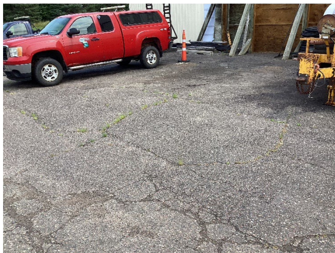
Failing Pavement
