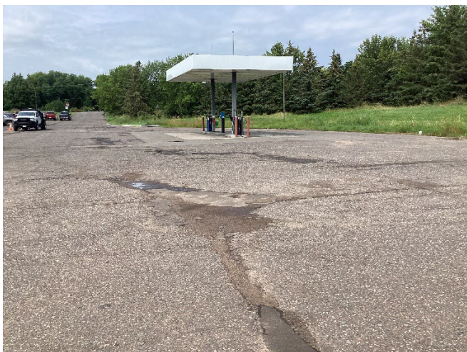
Failing Pavement
