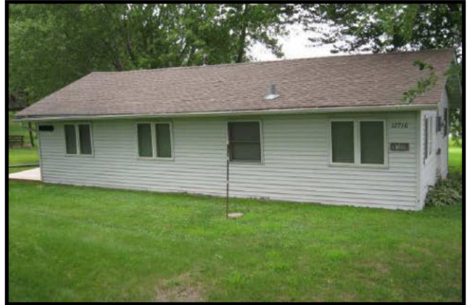
Photo taken in 2011; east wall (road side)
