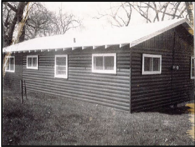
Photo taken in 1972; east wall (road side)
