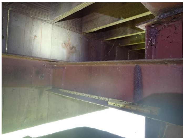
TYPICAL HORIZONTAL CANTILEVER CONNECTION
