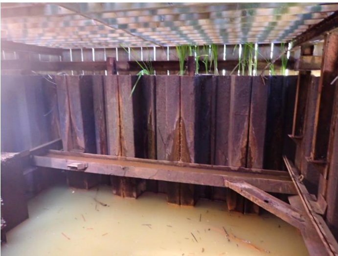
EAST SIDE OF CONTAINMENT CELL LOOKING EAST
