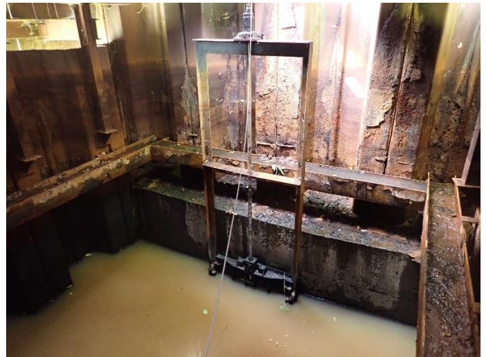
WEST SIDE OF CONTAINMENT CELL LOOKING WEST
