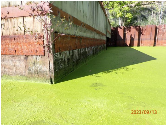
NORTH FACE OF WEIR LOOKING WEST
