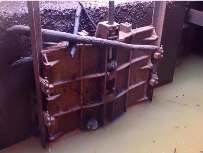
WEIR GATE CONDITION LOOKING NORTH
