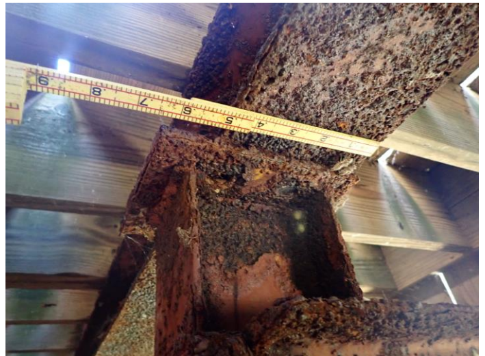
TYPICAL HORIZONTAL SUPPORT CONNECTION CONDITION
