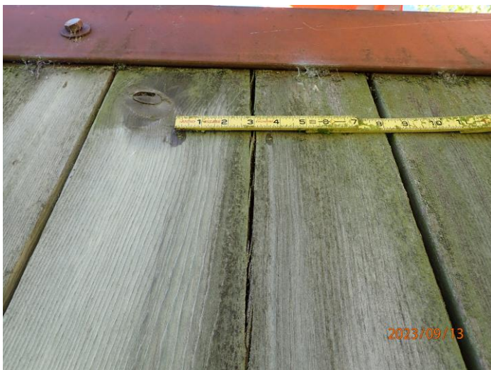
TYPICAL CHECKING OF VERTICAL TIMBER PLANKS
