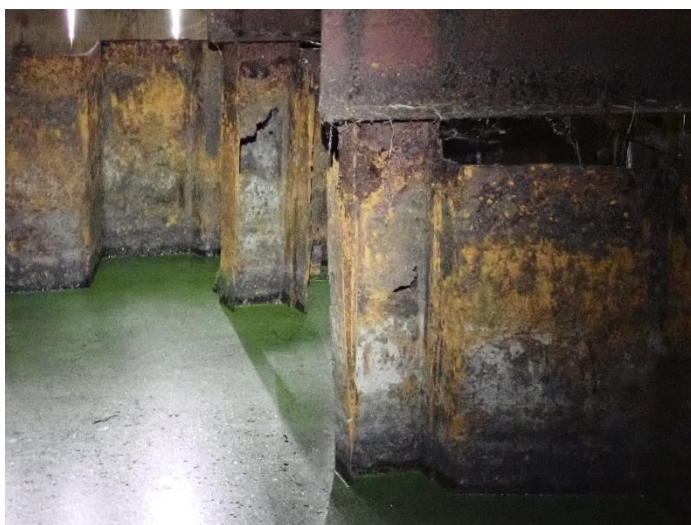
TYPICAL VERTICAL STEEL COLUMN CONDITION
