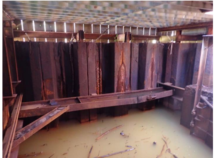
WEST SIDE OF CONTAINMENT CELL LOOKING WEST
