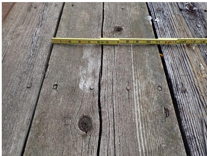
TYPICAL CHECKING OF WEIR DECK
