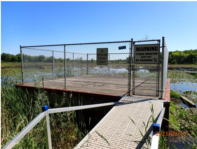
NORTH FACE OF WEIR LOOKING SOUTH
