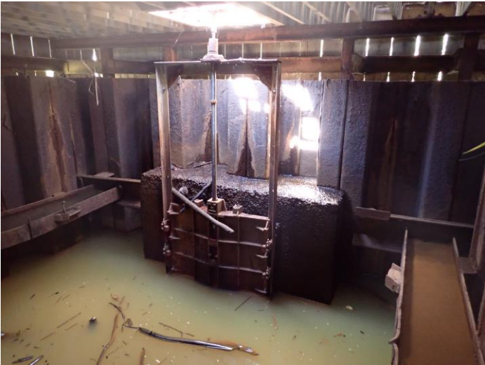
NORTH SIDE OF CONTAINMENT CELL LOOKING NORTH
