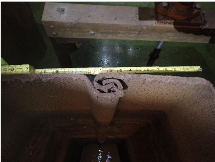
TYPICAL STEEL INTERLOCK CONDITION
