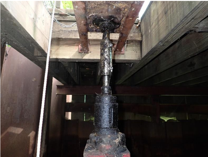
WEIR GATE LIFT CONDITION LOOKING NORTH
