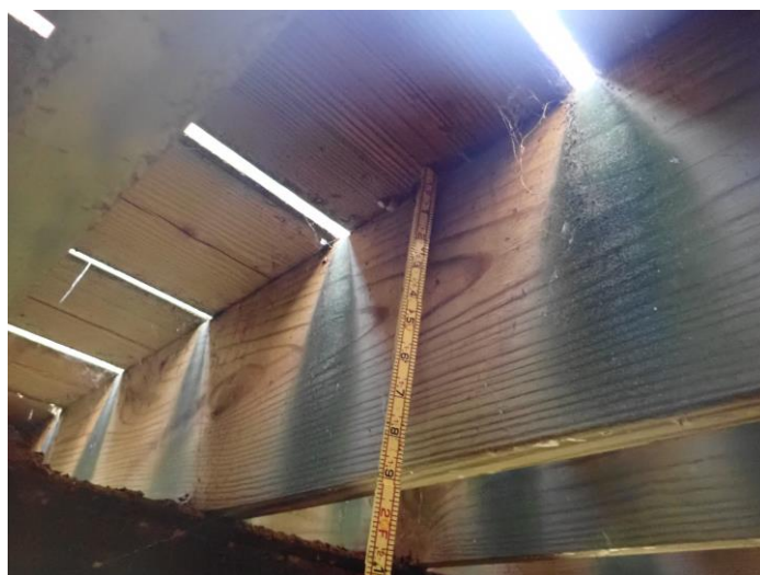
TYPICAL FLOOR JOIST CONDITION
