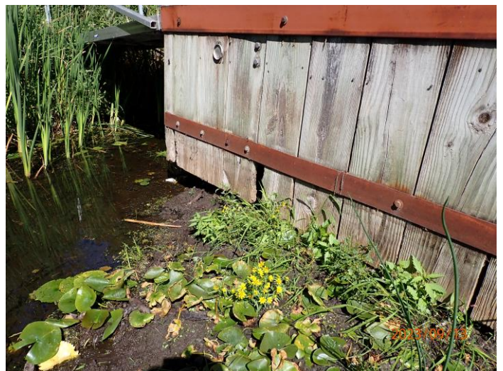
WEST FACE OF WEIR LOOKING NORTH
