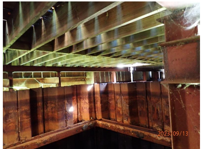
EAST SIDE OF CONTAINMENT CELL LOOKING NORTHEAST
