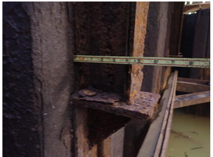
TYPICAL VERTICAL COLUMN CONDITION
