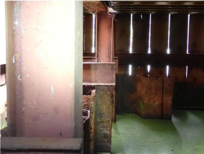
TYPICAL DEFLECTION OF STEEL COLUMNS
