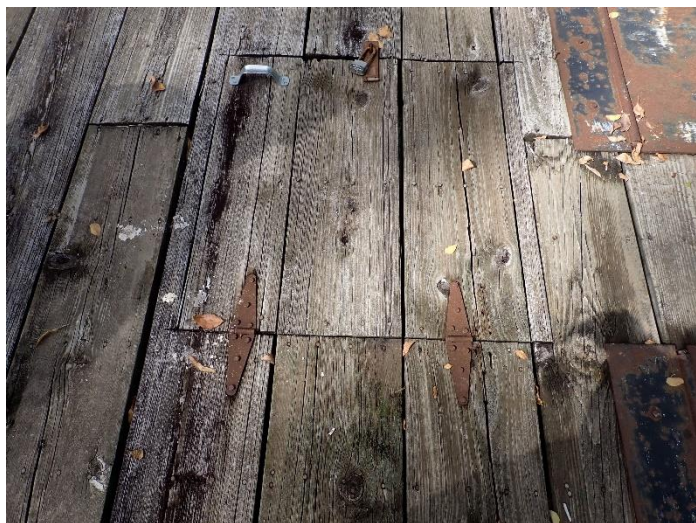
TYPICAL ACCESS HATCH CONDITION
