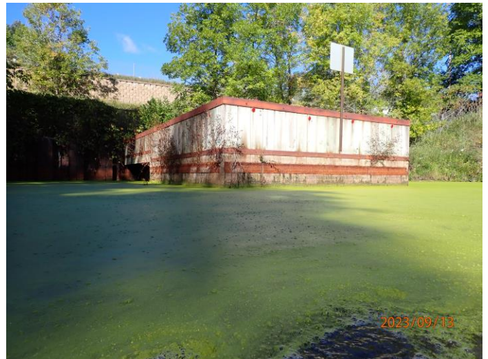
EAST FACE OF WEIR LOOKING NORTHWEST
