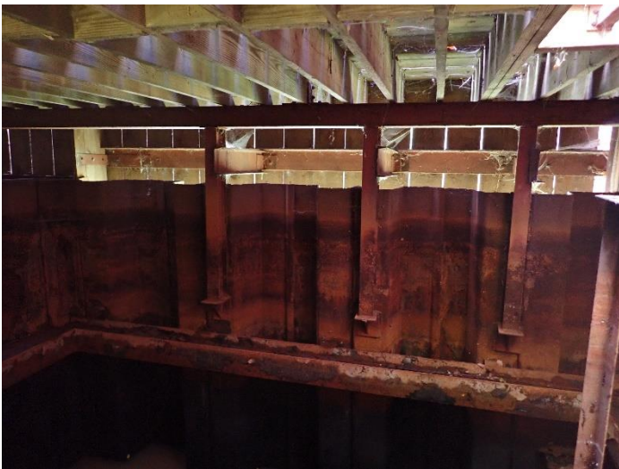
SOUTH SIDE OF CONTAINMENT CELL LOOKING SOUTH
