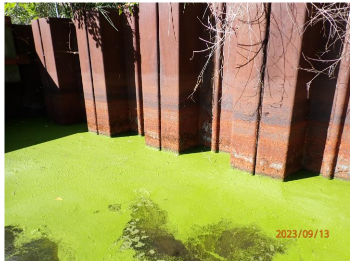
STEEL SHEET PILING ALONG THE WEST FACE OF WEIR LOOKING SOUTHWEST
