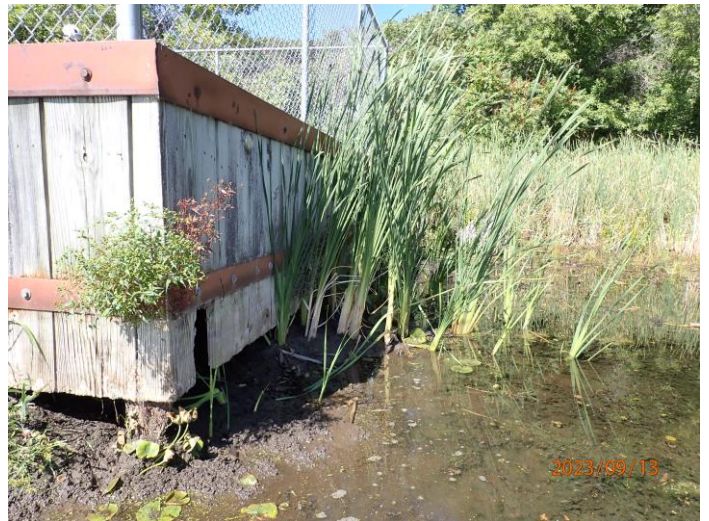
EAST FACE OF WEIR LOOKING NORTH
