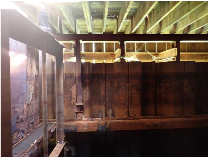
NORTH SIDE OF CONTAINMENT CELL LOOKING NORTH
