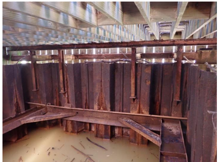
SOUTH SIDE OF CONTAINMENT CELL LOOKING SOUTH
