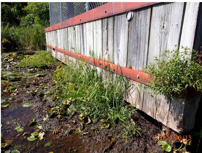
SOUTH FACE OF WEIR LOOKING NORTHWEST
