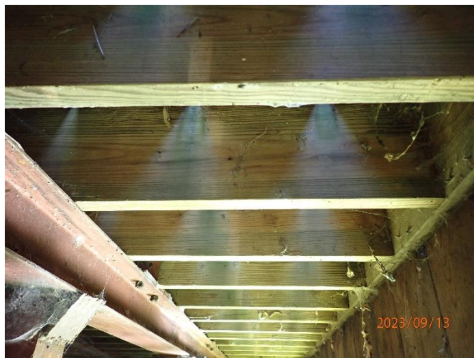
TYPICAL FLOOR JOIST CONDITION
