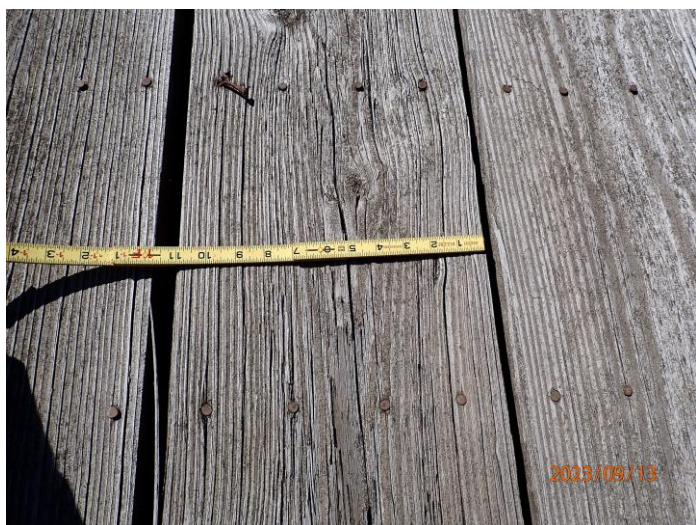
TYPICAL CHECKING OF WEIR DECK
