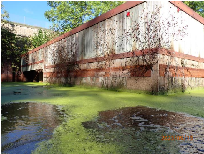
SOUTH FACE OF WEIR LOOKING NORTHWEST
