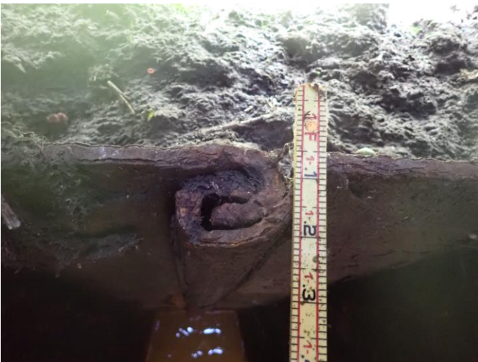
TYPICAL STEEL INTERLOCK CONDITION
