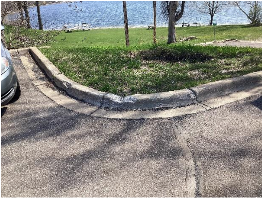
Damaged Curbing
