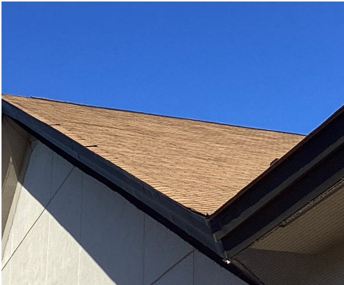
Roof beginning to show curling and lifting
