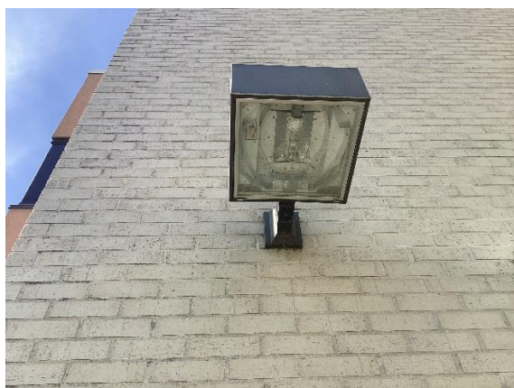
Old Exterior Lighting
