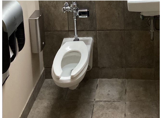
Damaged tile and missing tile grout
