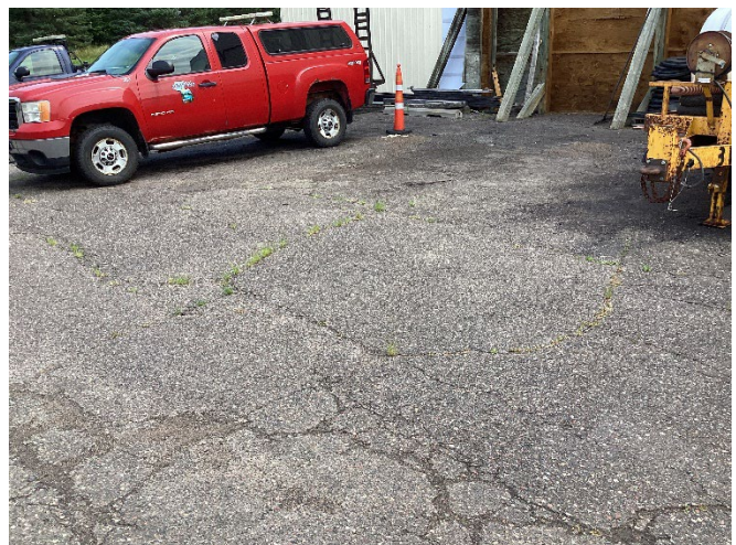
Failing Pavement
