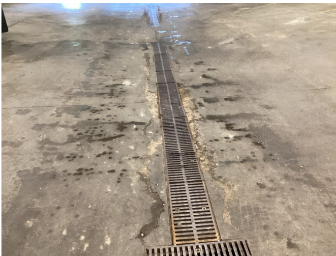
Damaged concrete in main shop
