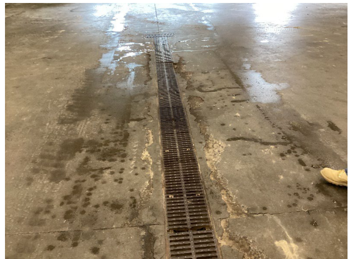
Damaged concrete in main shop
