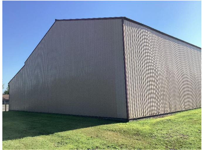
Bowing exterior walls
