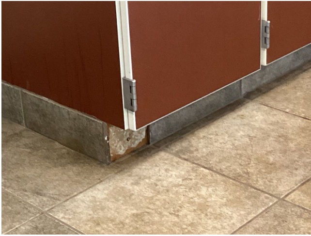
Damaged tile and missing tile grout
