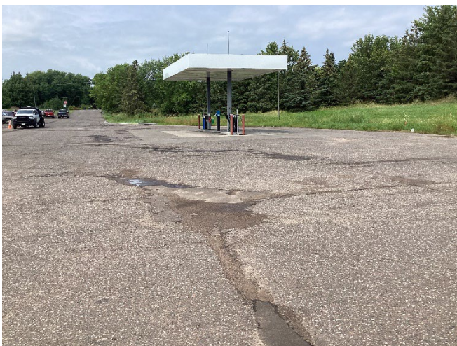
Failing Pavement
