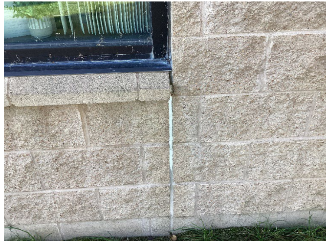
Dried and missing flexible sealants
